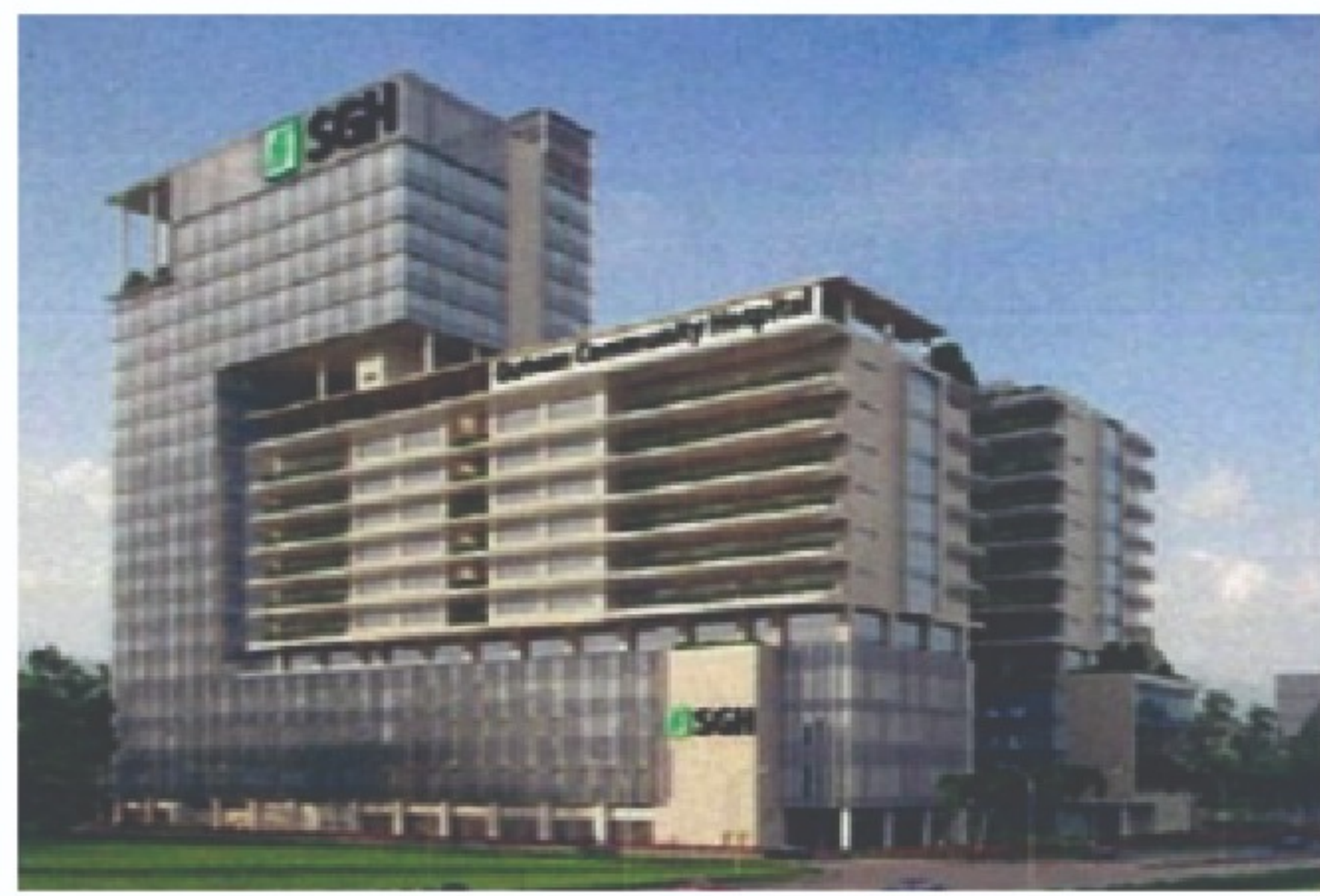
OCH Hospital Project Main Contractor - Penta Ocean Construction Pte Ltd Our Client - Yongnam Engineering Pte Ltd
